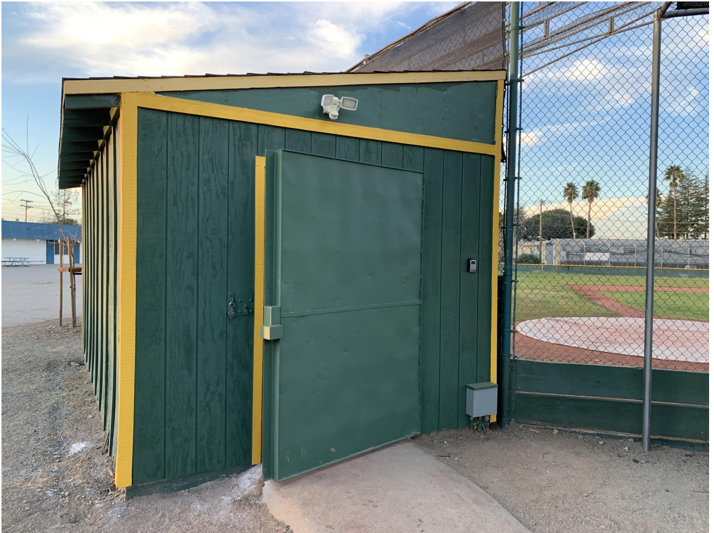
Major Shed Door Repairs
